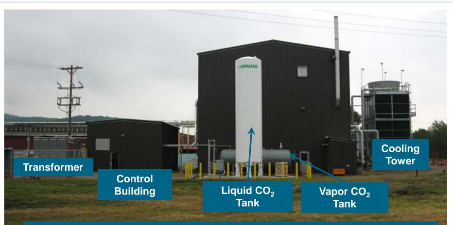
In parallel with the Gen1 design efforts, a new 10 MW, 2,200 PSI test facility was designed and built on the Olean, NY campus.
